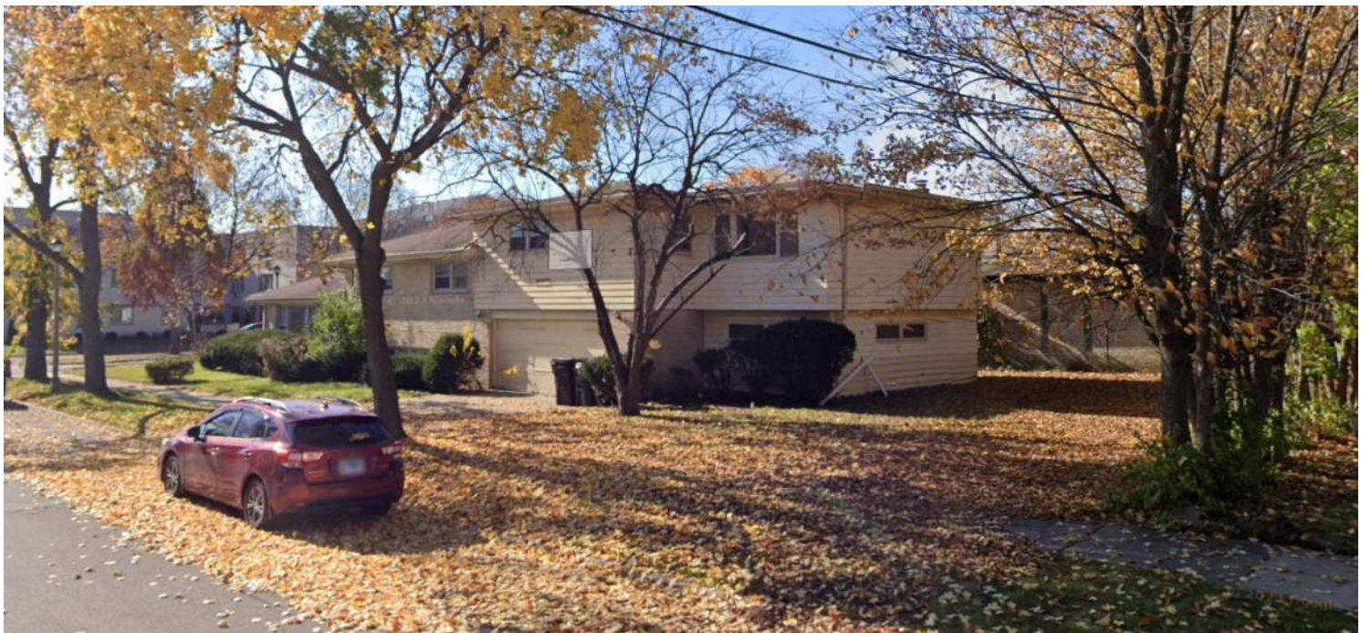
EXISTING NORTHEAST VIEW
