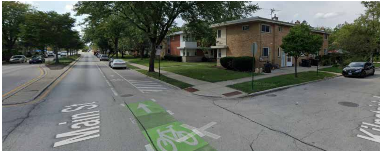
B Looking from SW corner of site down Main St and Kilpatrick Ave
