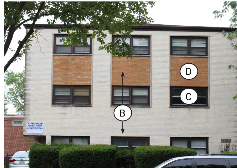
BUILDING ALONG MAIN STREET (4700 BLOCK)
