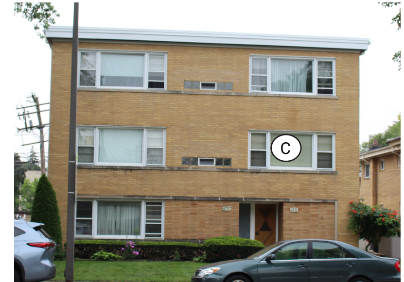
BUILDING ALONG MAIN STREET (4700 BLOCK)
