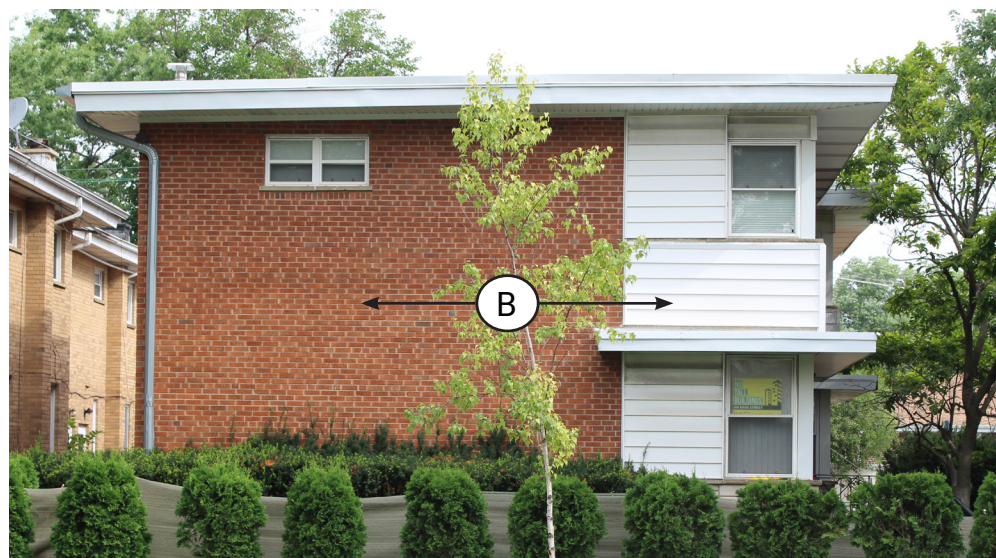
BUILDING ALONG MAIN STREET (4700 BLOCK)
