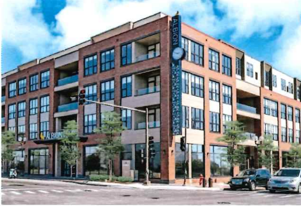
Figure 4 The 161-unit Albion at Renaissance Place on Green Bay Road in Highland Park was approved in 2020 and offers 27 inclusionary units for households with incomes between 45-100% of the area median income.
