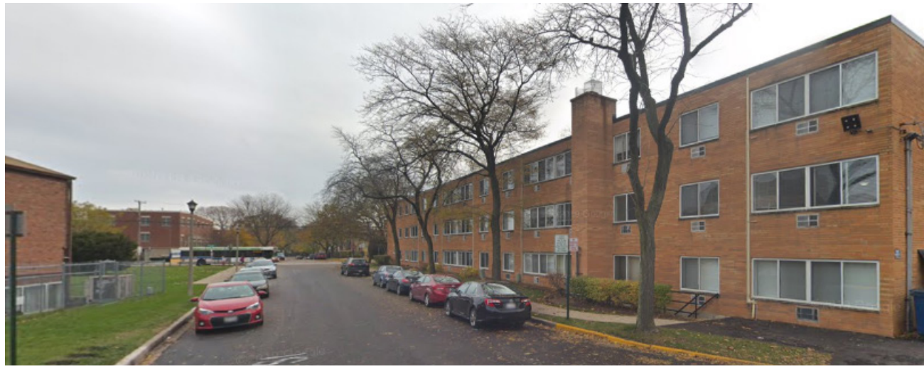
A SW corner of Site from Greenleaf St
